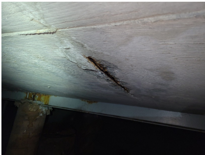
Photograph #4 – Rust and spalling in concrete slab reinforcement and concrete slab.
