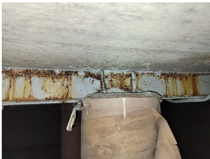
Photograph #2 – Steel beams with lower severity of rust damage.
