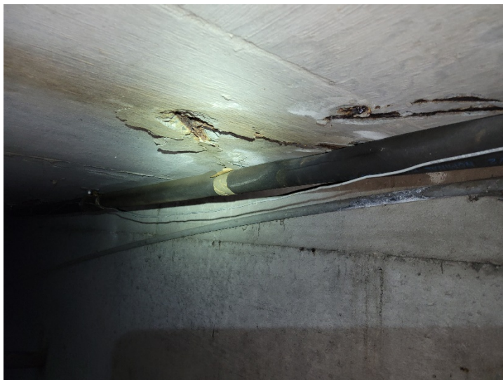
Photograph #5 – Spalling and slab damage
