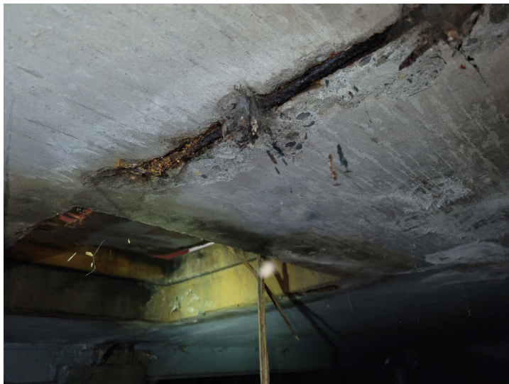
Photograph #3 – Severe rust and spalling in concrete slab reinforcement and concrete slab.
