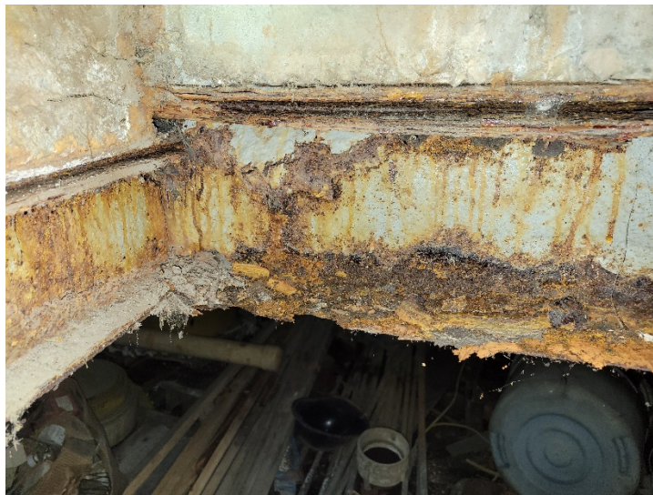
Photograph #1 – Steel beam with missing bottom flange and severe rust.
